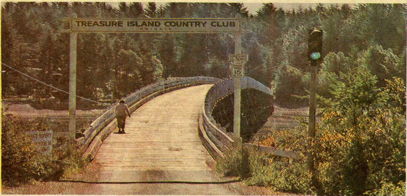
Staff photo by Bob Rudsit Traffic light signals the old bridge will go
